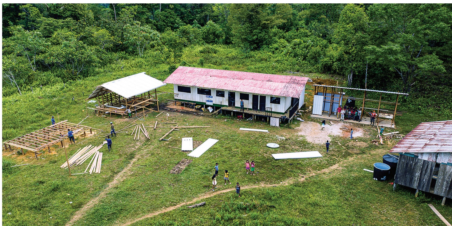
📷 Renovation of damaged school in indigenous community in Antioquia, Colombia
