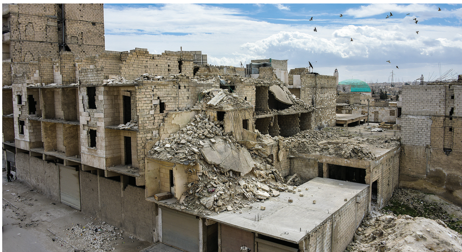
📷 Buildings in Aleppo, Syria damaged by the 2023 earthquakes
