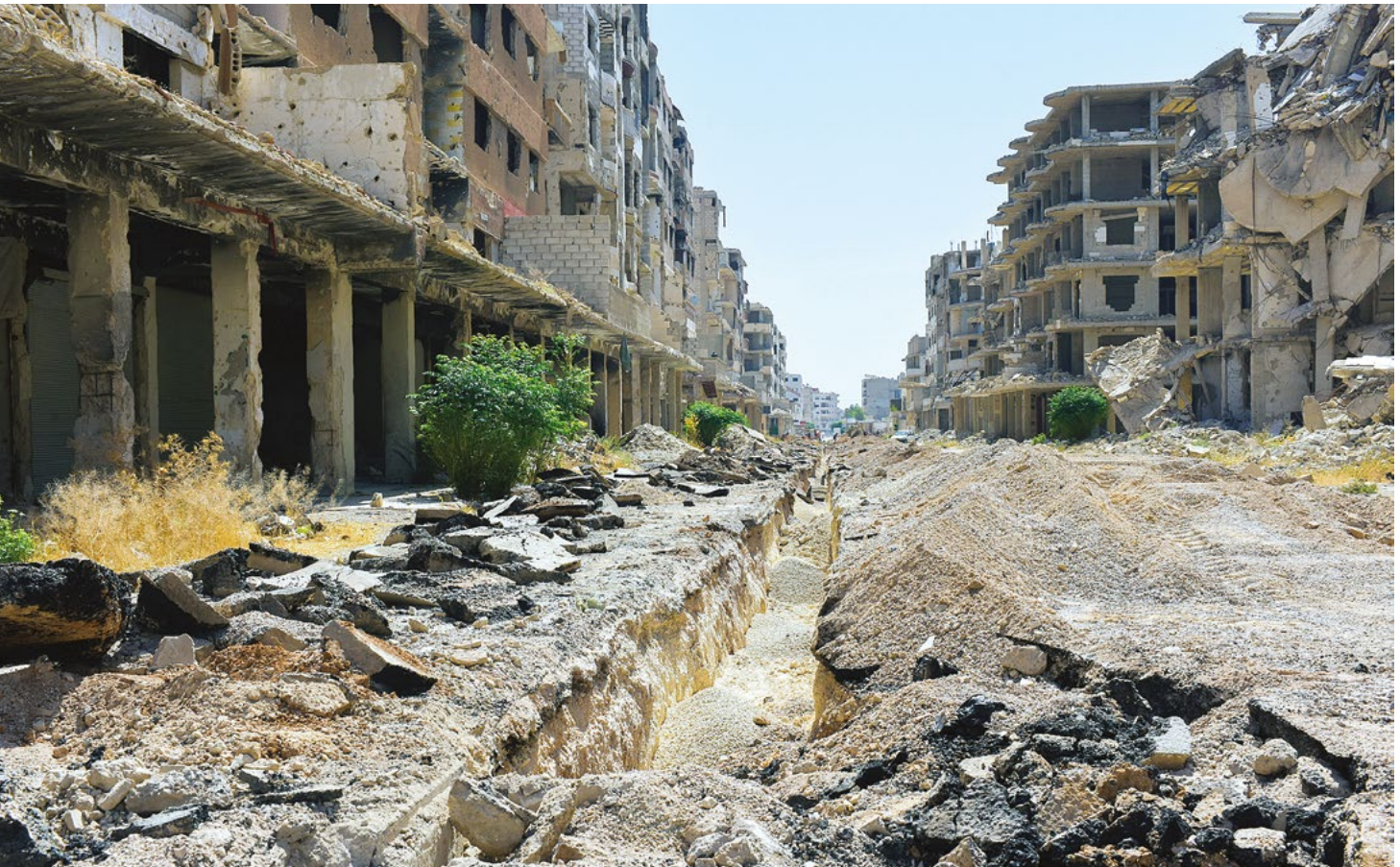
📷 Water system rehabilitation in Daraya, Rural Damascus, Syria
